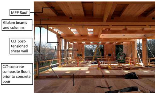
Fig. 2. Depiction of materials used in the George W. Peavy Forest Science Complex.
